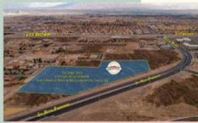
An aerial view of the property where the Southwest Water Reclamation Facility will be built.
